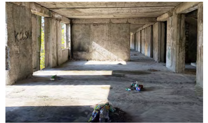
Interior view, Big Sori
