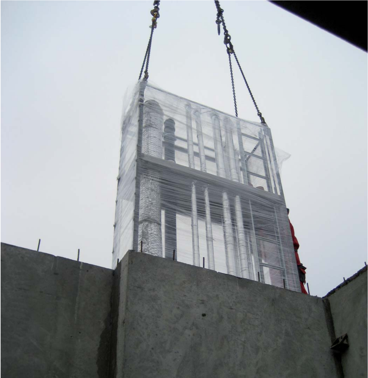
The shaft is lifted into place, Photo: NCC Construction DK
