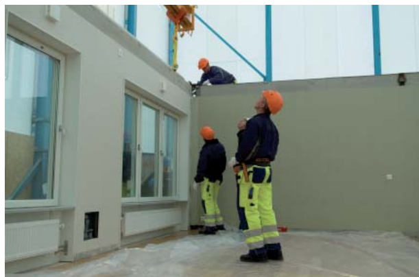
NCC Komplet, Assembly on site. Photo: NCC AB
