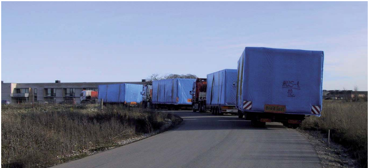
Units are transported to the building site on trucks. Photo: Tegnestuen Vandkunsten
