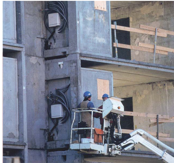
Pods are installed in a multi-storey building
