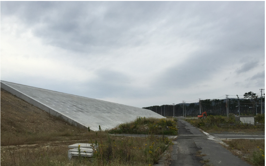
Seawall under construction, 7,4 meters high. Watanoha District.
