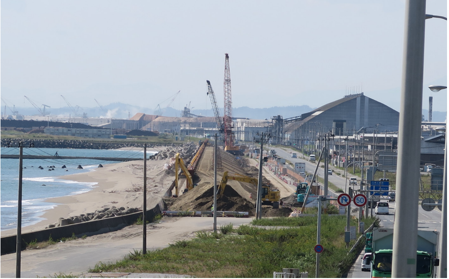
Seawall under construction, 8,4 meters high Ishinomaki.
