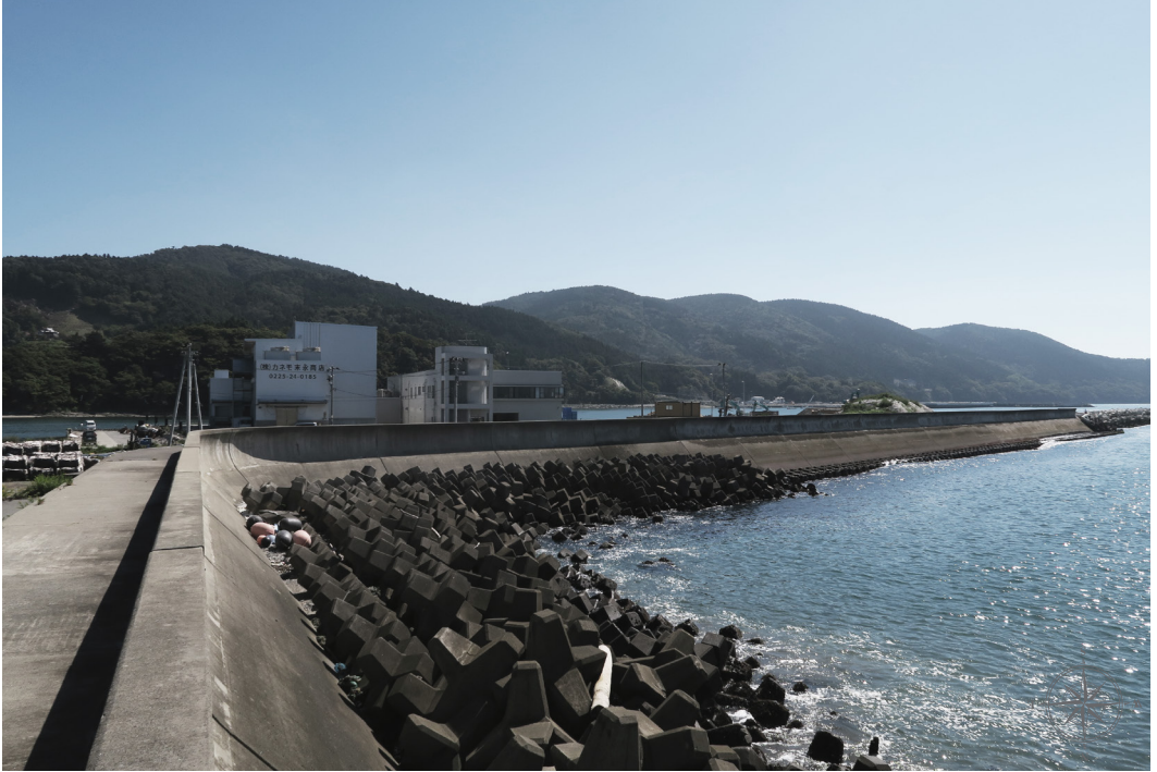
View from the west, the old seawall and site. The hilly peninsula in the background.
