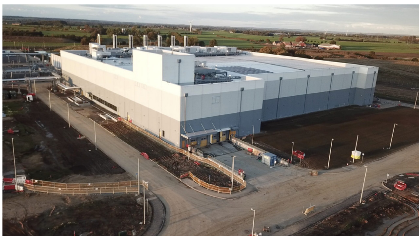
Google datacenter, Fredericia
