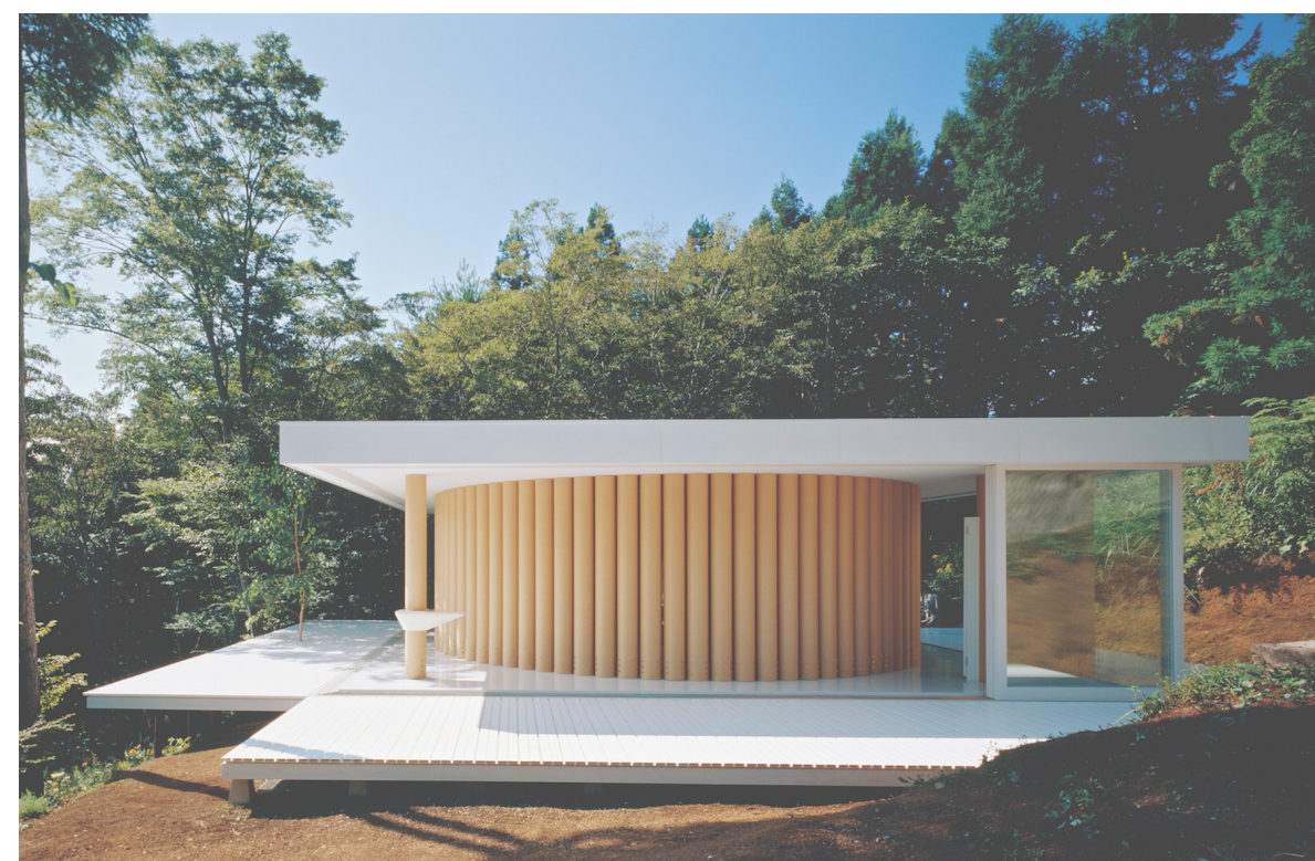
SHIGERU BAN / Paper House This was the first project in which paper tubes were authorized for use as a structural basis in a permanent building.
