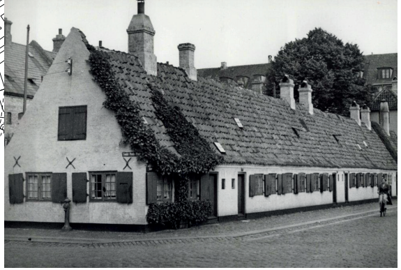
Figure 12: Original Nyboder housing structure, 1936
