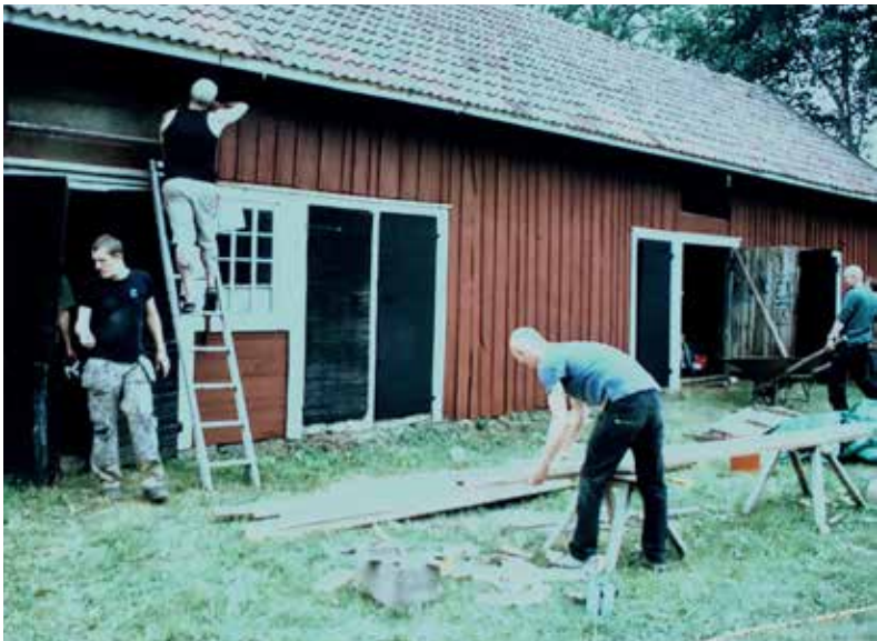
Picture looking south-west at the small barn. Maintenance work 2010.
