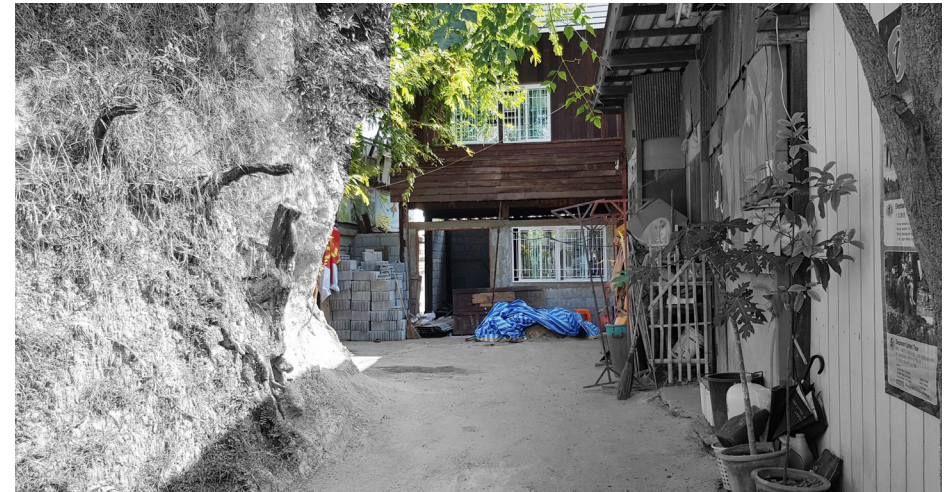
The image from the street side depicts how the house is hidden behind the earthen wall.
