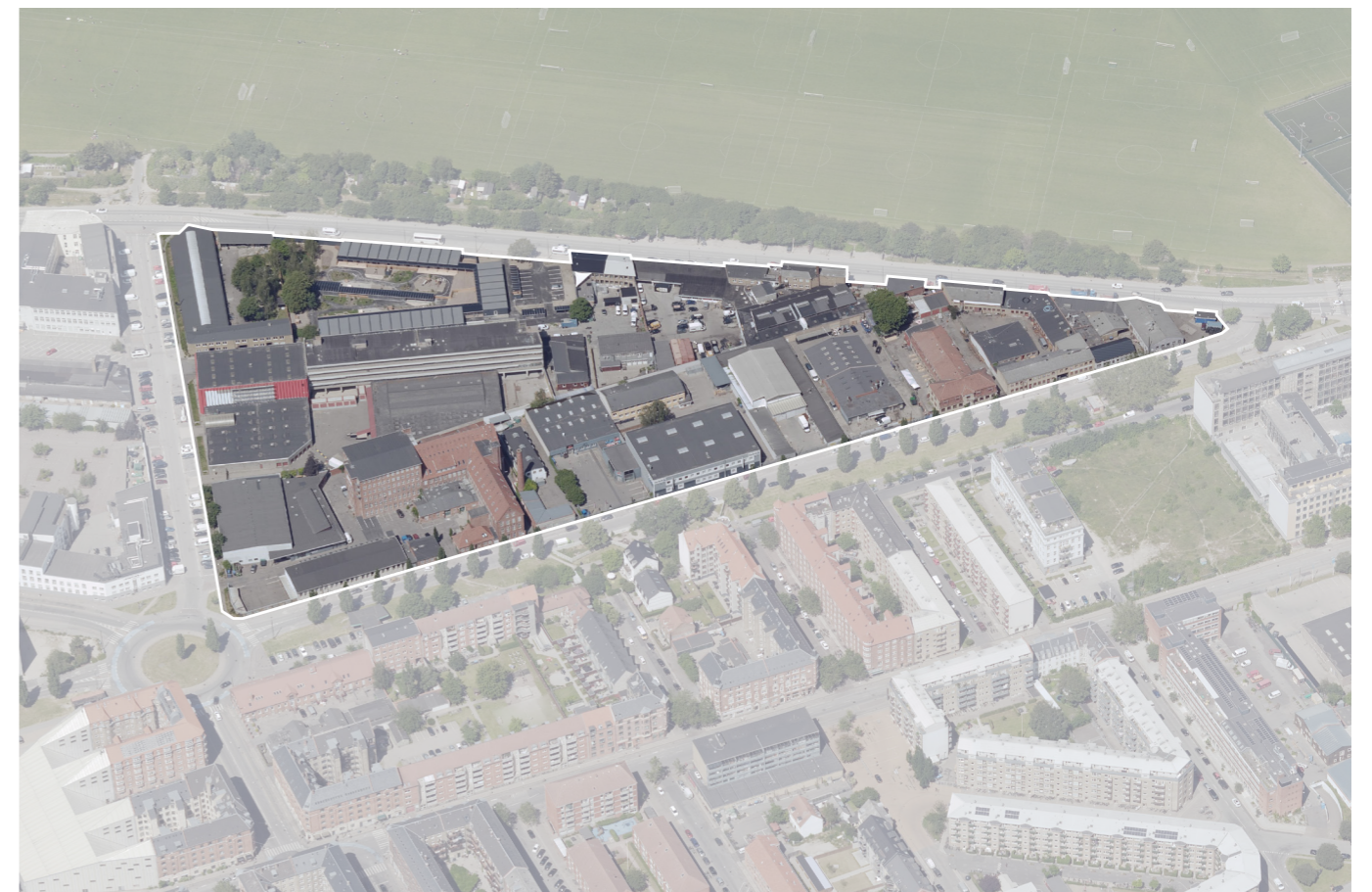
Figure 7: Zoom in on the site seen from the North
