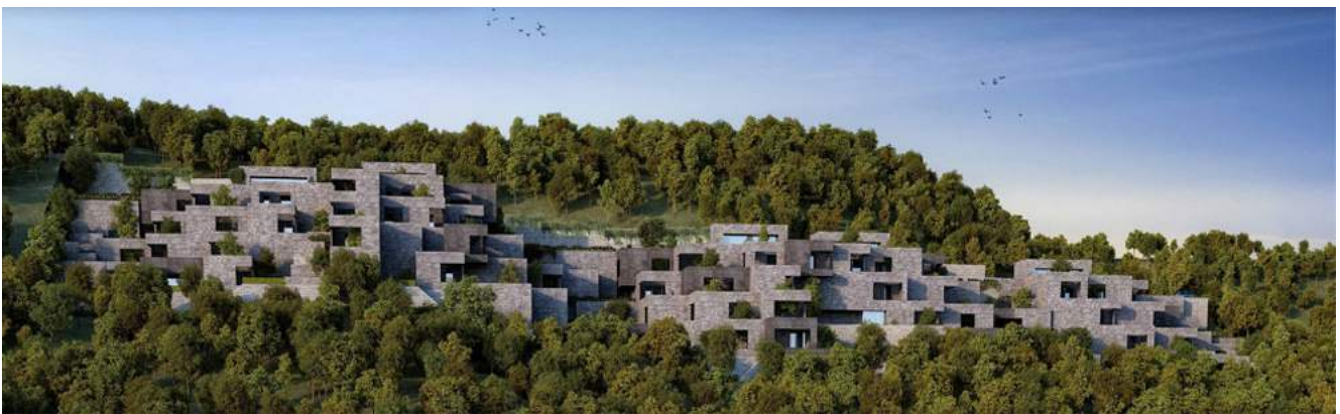
The Village by Sunjay Puri Architects
