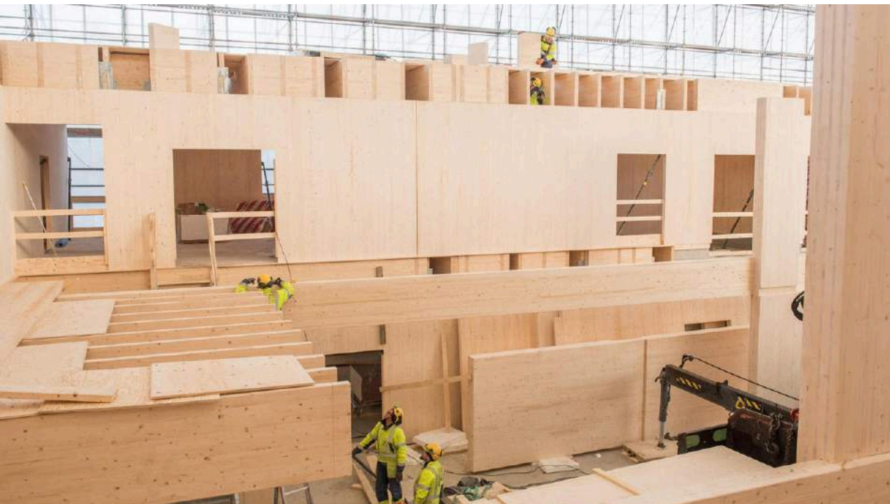
Cross laminated timber construction
