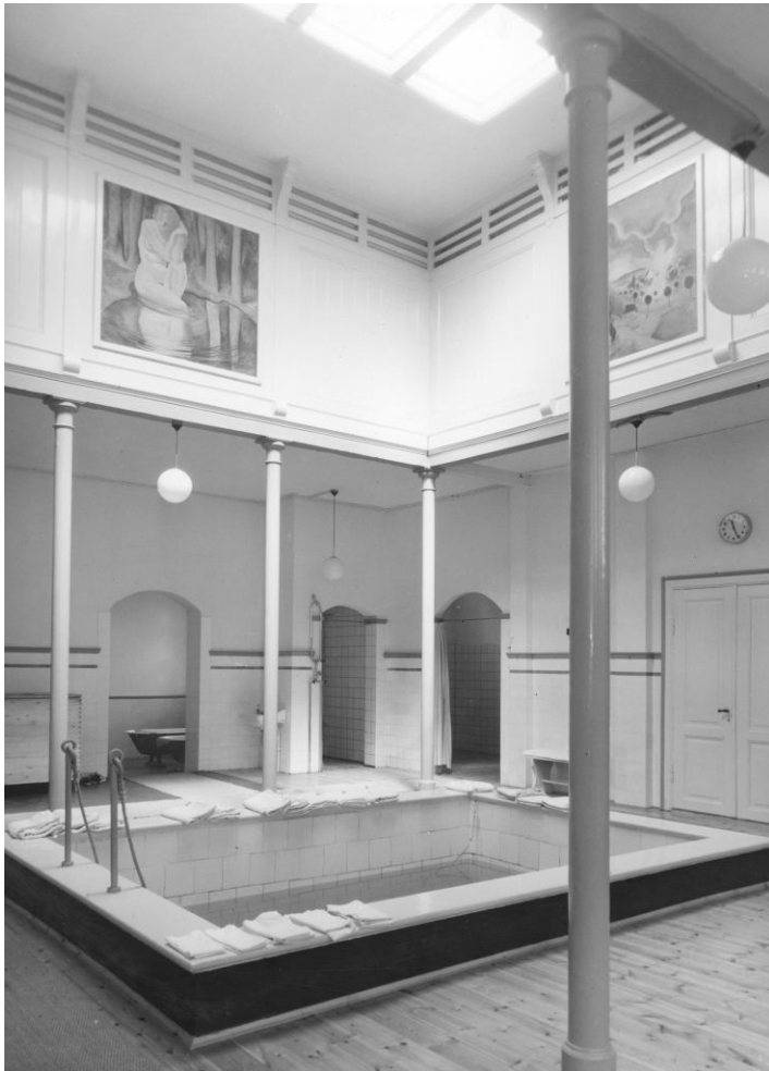
Silkeborg Vandkuranstalt designed by Vilhelm Dahlerup, 1883
