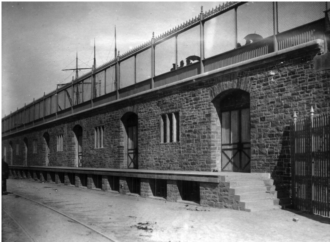
Langelineskuret seen from the western side showing the railway, fenced promenade on the roof and the masts from ships docking in the background. 14/9-1894. kbhbilleder.dk
