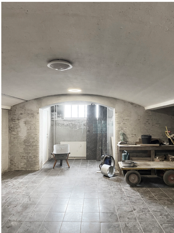
The arched frames and the clerestory windows in the basement
