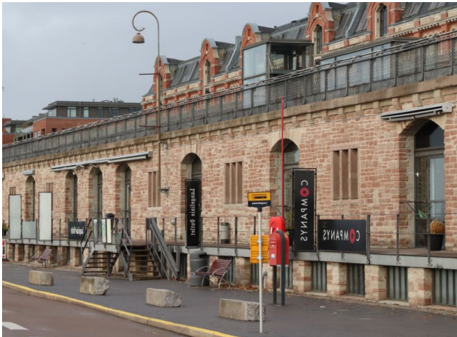
Langelineskuret in present time with outlet signs and bus stops
