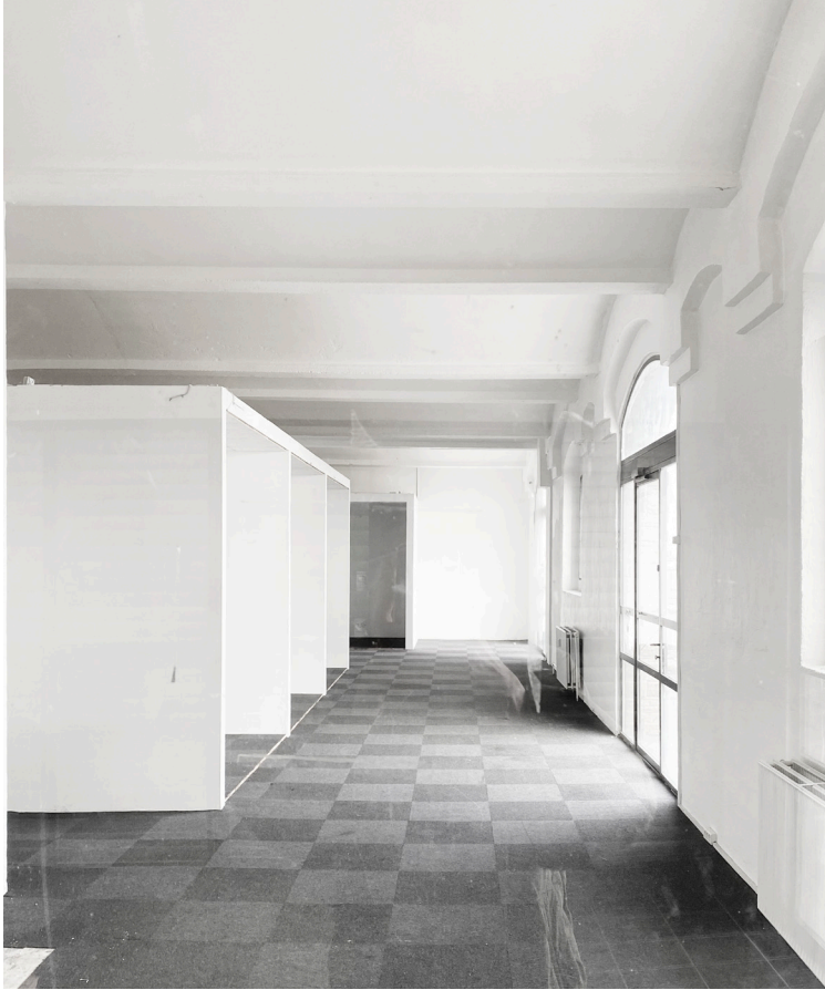
An empty area on the groundfloor with split into smaller tenancies by flexible walls
