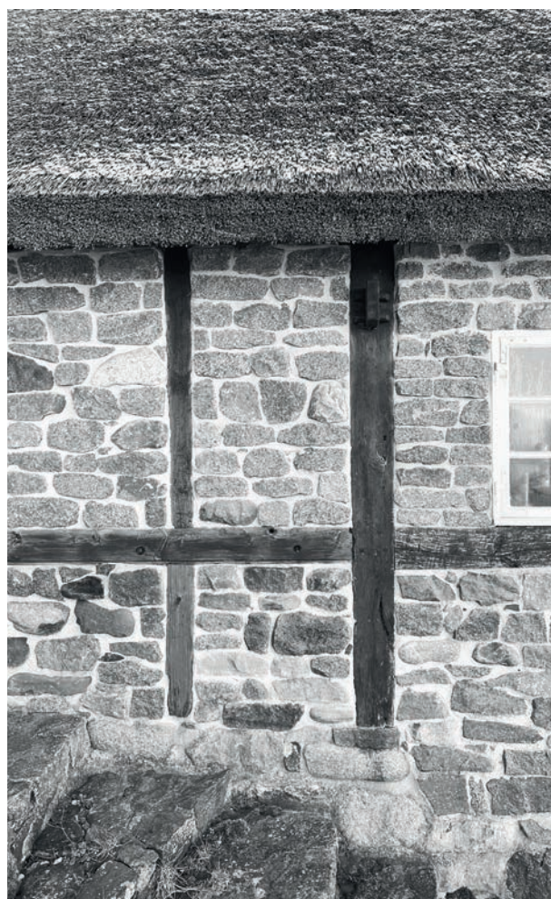
Details and timber frames
