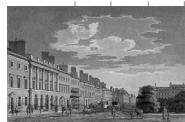
Grosvenors Square, London (1727) Robert Adam Great Fire of London Note: not affordable but credited with the start of the terraced typology and building standards
