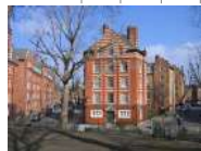
Boundary Estate, London (1890-1900) LCC under Owen Fleming. Considered the worlds first council estate. Arts and Craft aesthetic. Clearing of the slums
