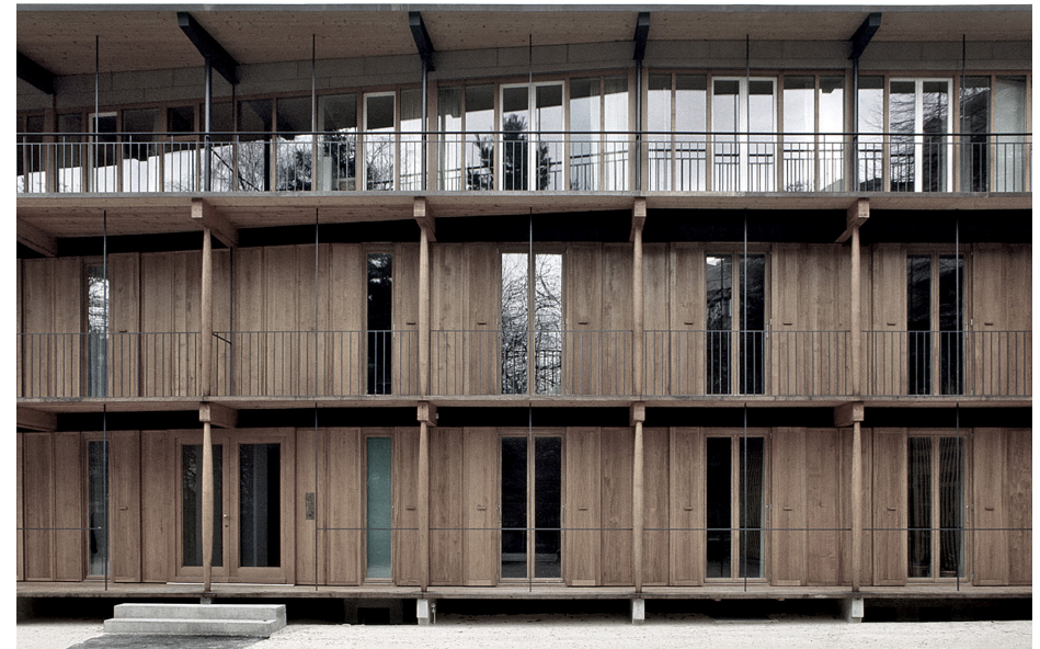
Apartment Building along a Party Wall - Herzog & de Meuron Opført i 1988
