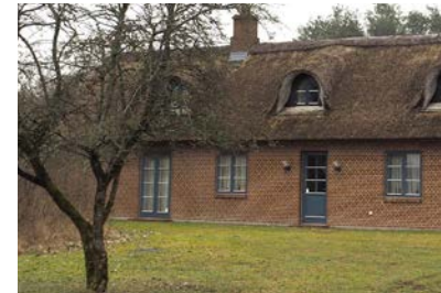
Figure 25. Photography of Hangarhuset , by author
