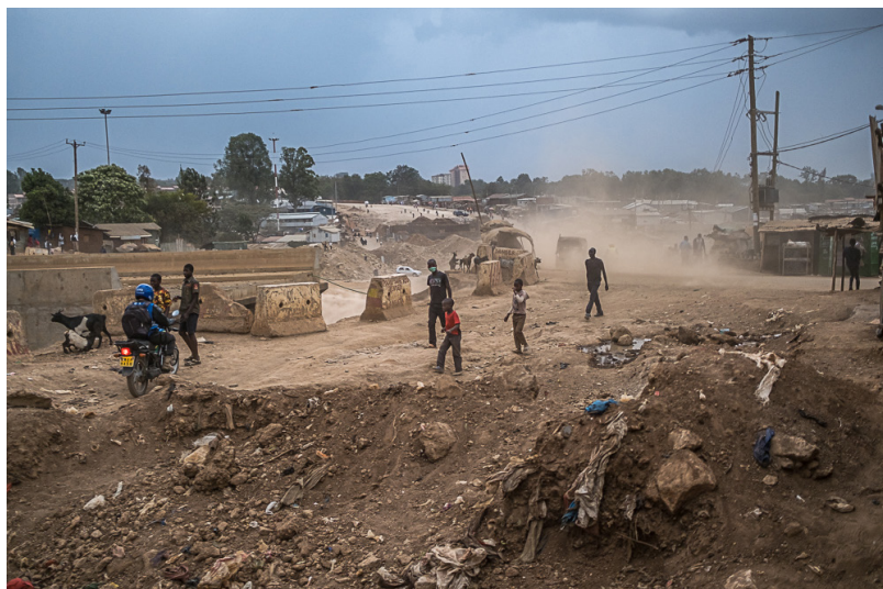
↑ The road as a construction site in Kibera (Brian Otieno)
