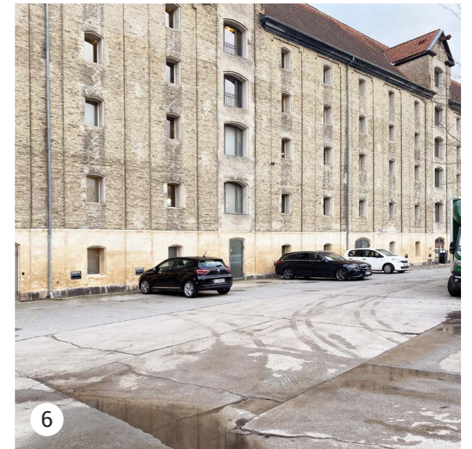
Behind food market, parking lot and broken asphalt
