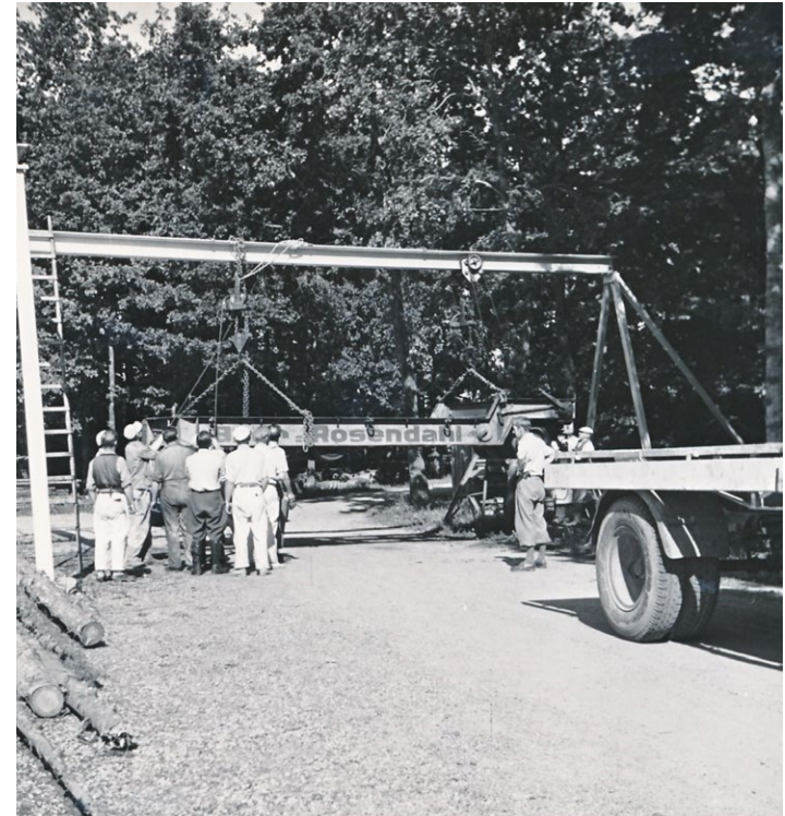
Fig. 19. Gjorslev Savvaerk in construction, 1950
