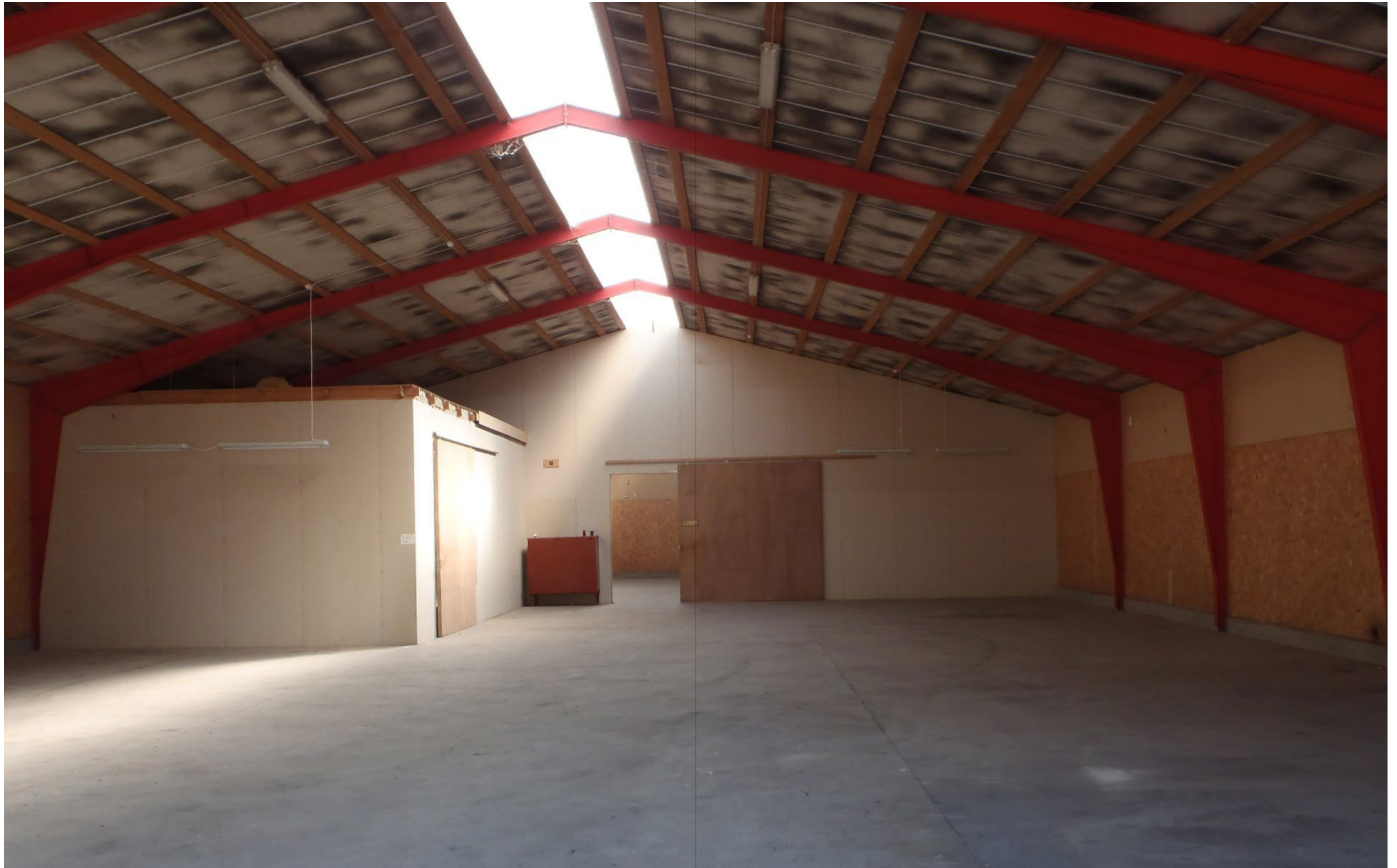
Fig. 26. Current state of interior of former workshop building
