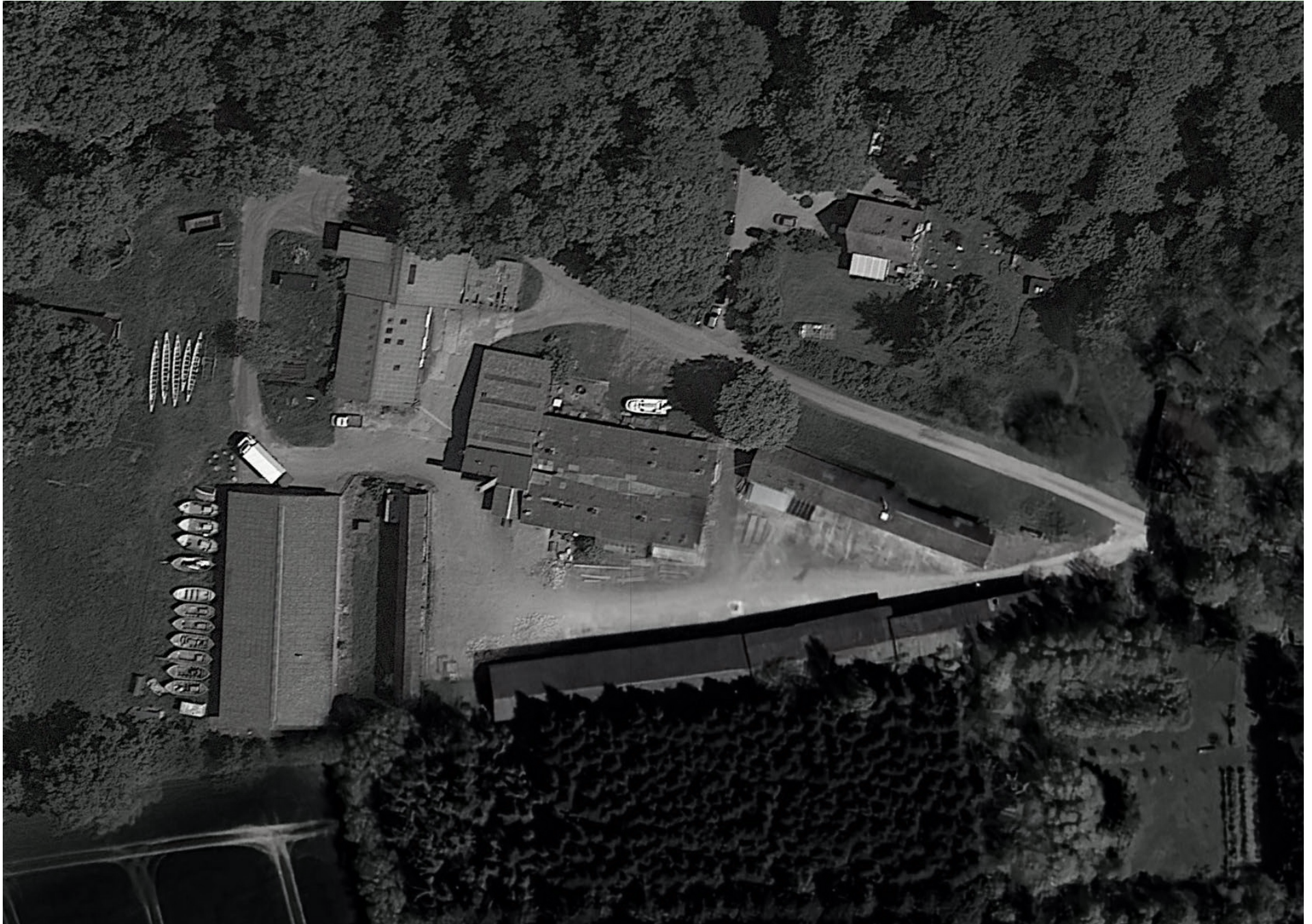
Fig. 12. Aerial view of site
