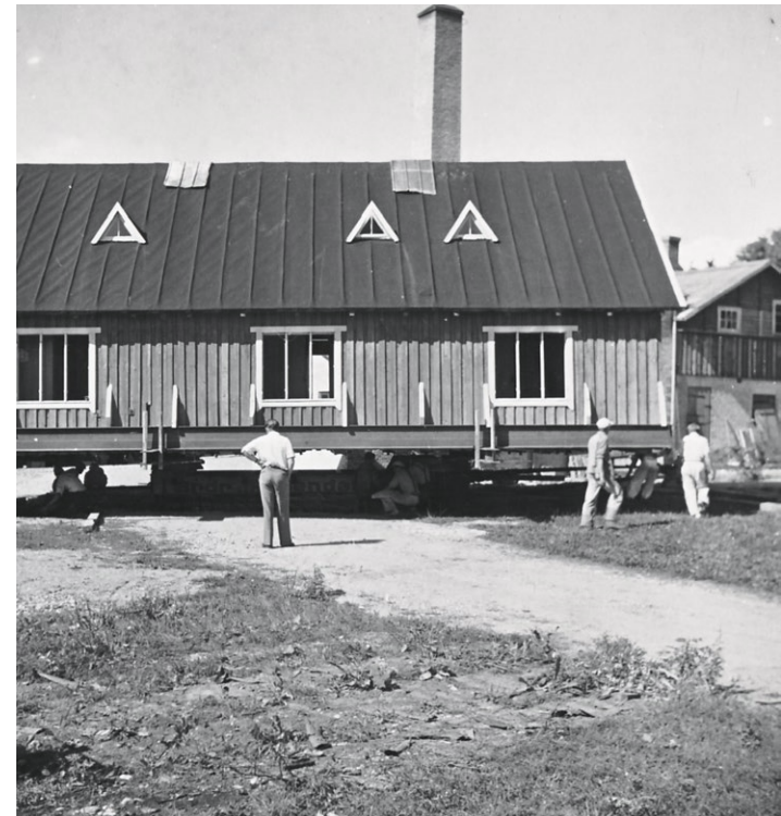
Fig. 17. Gjorslev Savvaerk in construction, 1950
