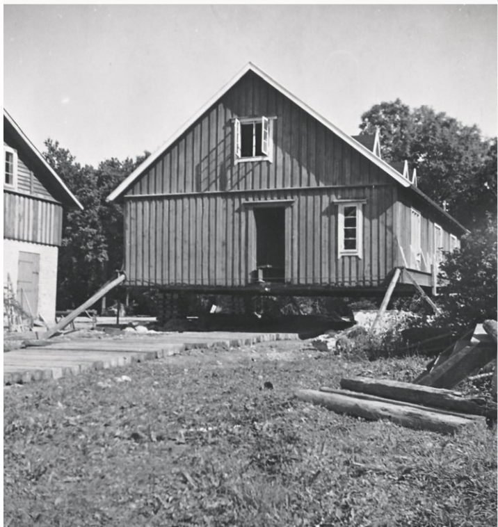
Fig. 16. Gjorslev Savvaerk in construction, 1950
