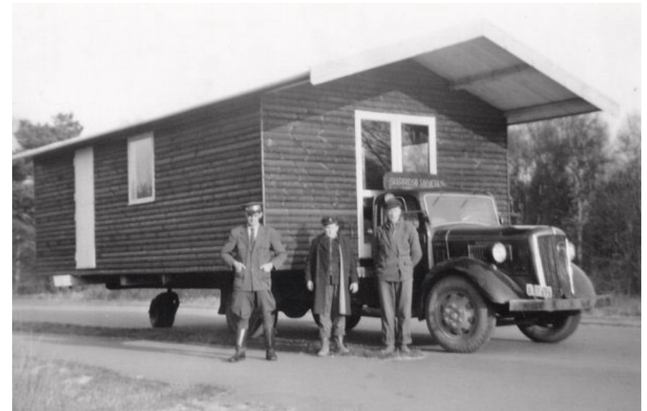
Fig. 63. A typical summer house from Skarridso Sawmill is on a block wagon on its way to its planned destination in the 1950s summer house landscape
