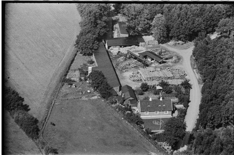
Fig. 13. Gjorslev Savvaerk in construction, 1950
