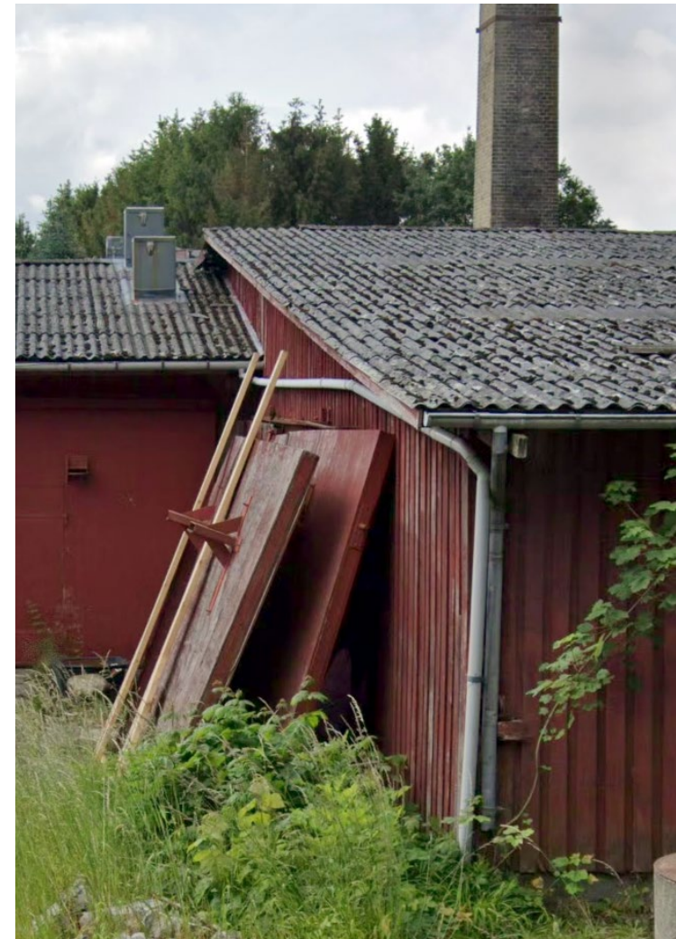
Fig. 40. Photo of site
