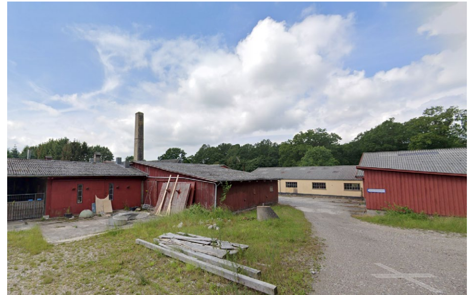
Fig. 23. Main driveway into site
