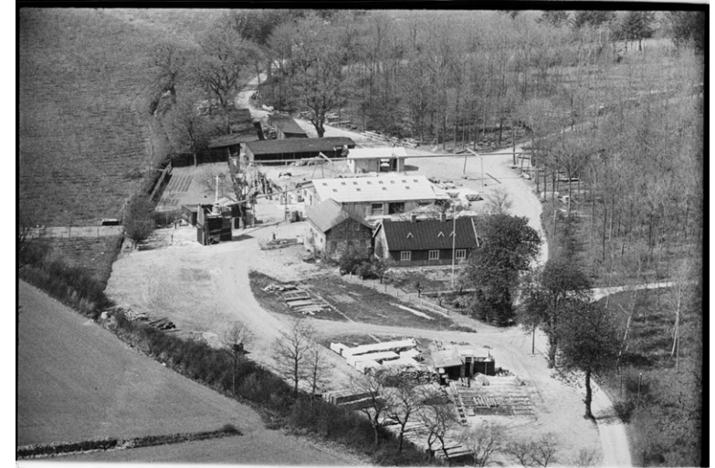
Fig. 14. Gjorslev Savvaerk in construction, 1950
