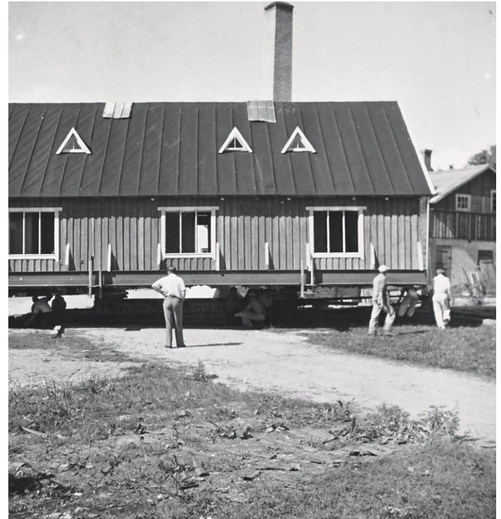
Fig. 16. Gjorslev Savvaerk in construction, 1950
