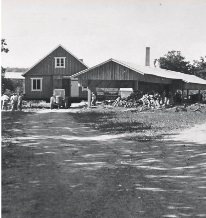
Fig. 17. Gjorslev Savvaerk in construction, 1950
