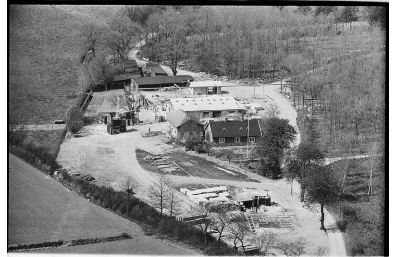
Fig. 13. Gjorslev Savvaerk in construction, 1950
