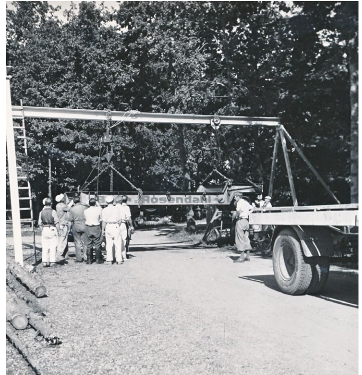
Fig. 18. Gjorslev Savvaerk in construction, 1950
