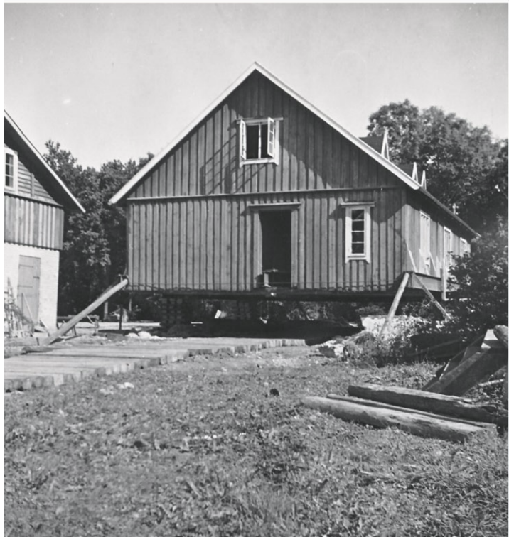
Fig. 15. Gjorslev Savvaerk in construction, 1950
