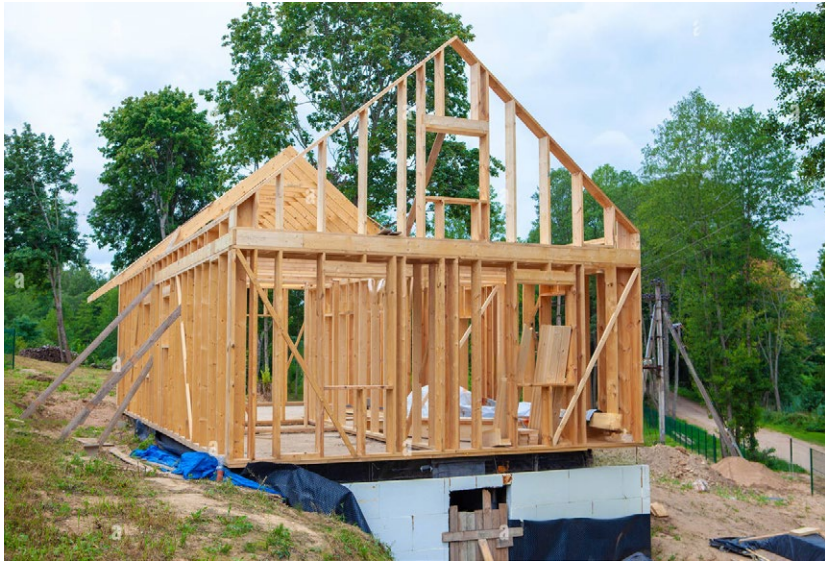
Fig. 33. Stick frame home under construction
