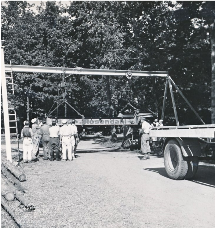
Fig. 40. Gjorslev Savvaerk in construction, 1950
