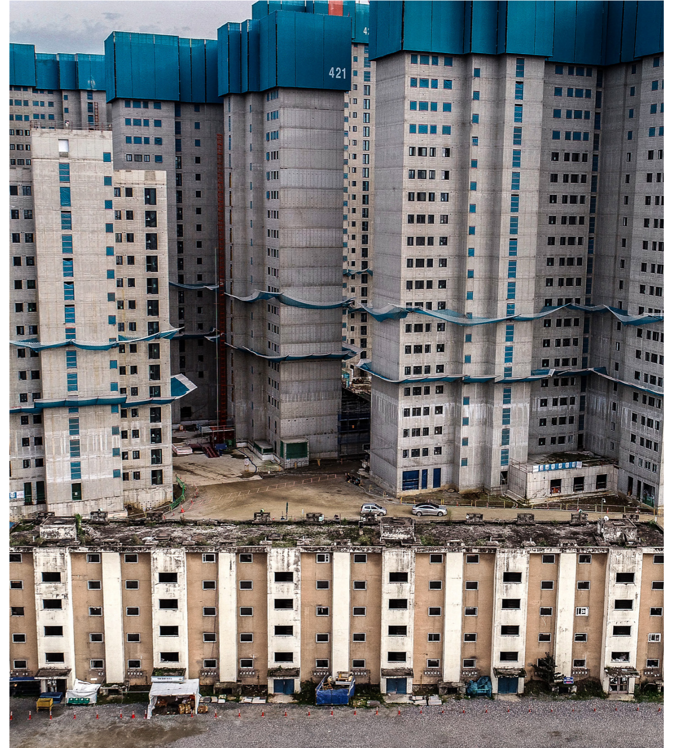
Fig01. An apartment reconstruction site in Seoul
