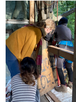
helping with tree house building
