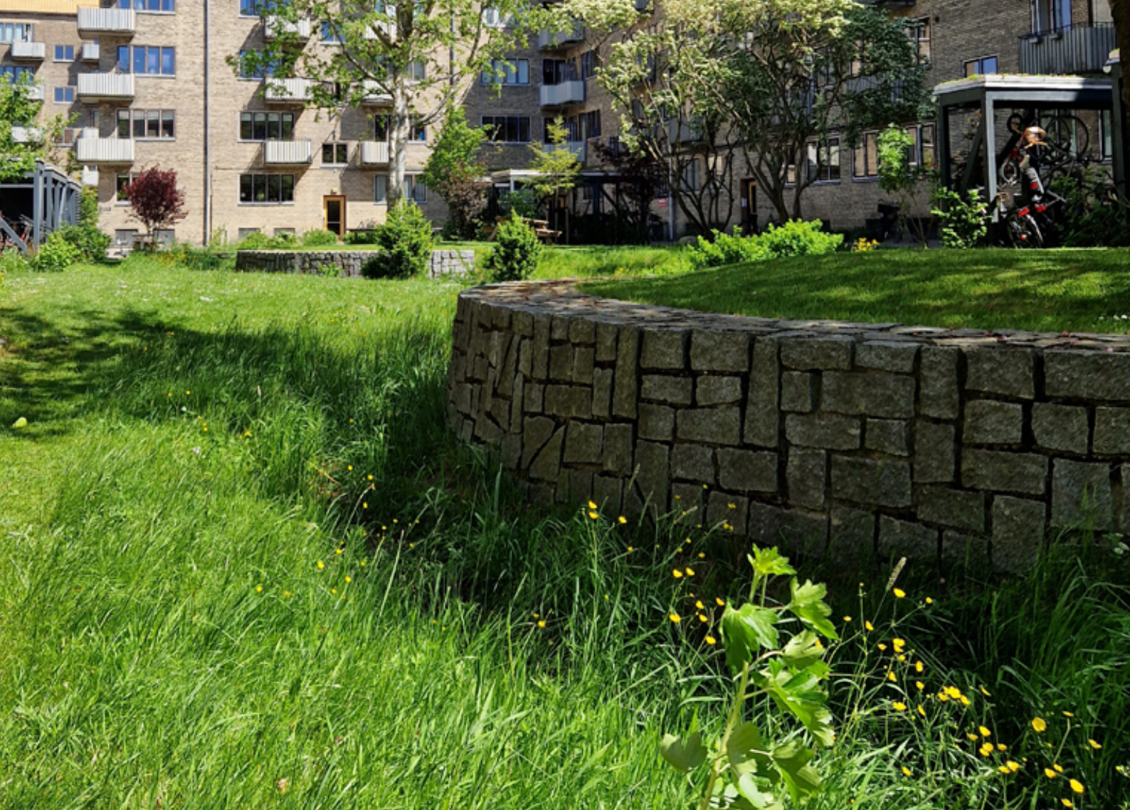
The trenches and ditches that utilise the landscape at The Courtyard of the Future at Askøgade by Niels Lützen Landscape Architects, KUBEN Management, Labland, Envidan, and UiWE (2020). photo by Emil Dencher, 2024.
