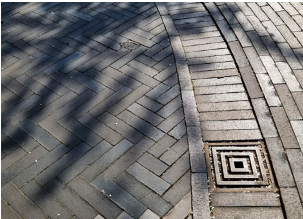
Trench made as a subtle incision into the pavement at Carlsberg Byen by 1:1 Landskab (2017). photo by Emil Dencher, 2024.
