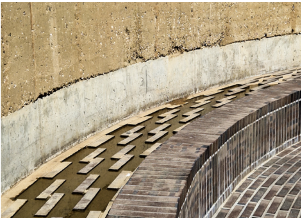
Brick trickling stairs inside the trench at The Courtyard of the Future at Tomsgårdsvej by SLA, NIRAS (2022). photo by Emil Dencher, 2024.
