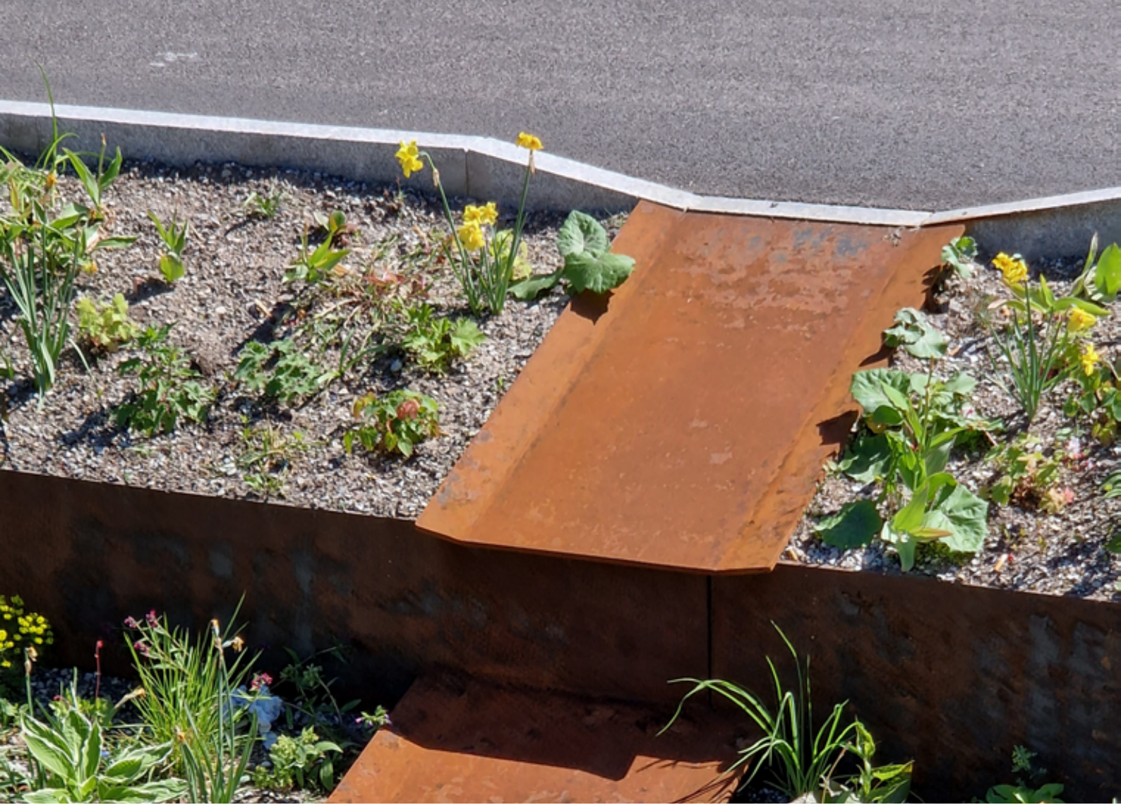
A trench as creating an outlet for rainwater detained on the road at Vibevej by Schønherr and Rambøll (2024). photo by Emil Dencher, 2024.
