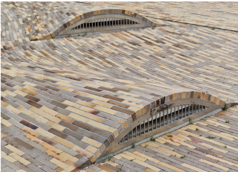
Distribution outlets into the brick riverbed at Karens Minde Aksen by Schønherr (2023). photo by Emil Dencher, 2024.
