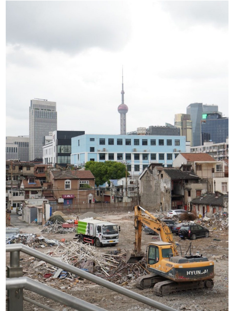
Fig 1. Demolition near Laoximen.
