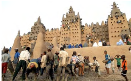
Figure 1 - Yearly re-plastering of the Grand Mosque of Djenné (source: Peter Howard - African World Heritage Sites).
