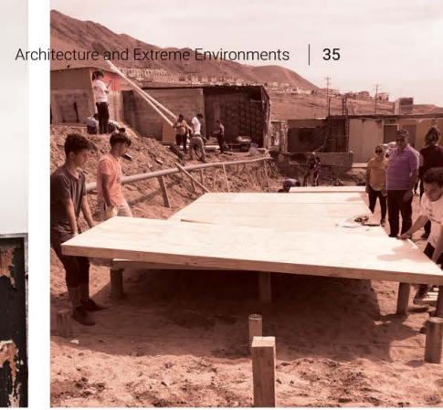
Rebuilding Campamento after Fire Fig 13
