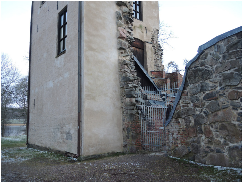
The northern tower
