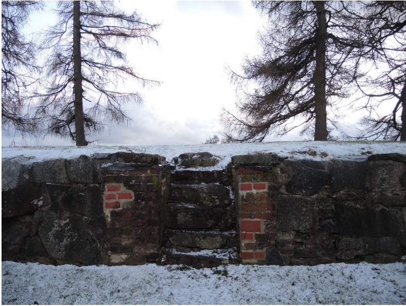
The eastern wall of the courtyard
