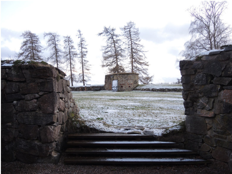
In the remains of the western tower, looking at the southern tower
