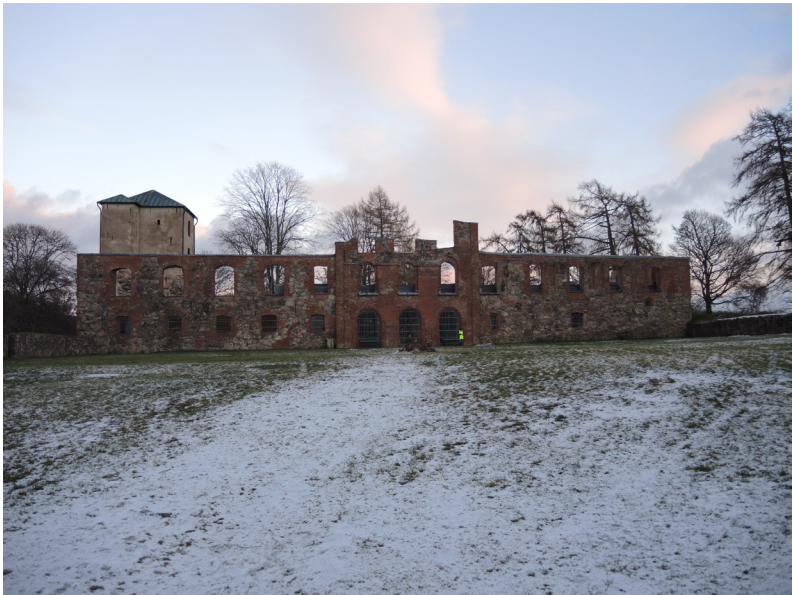
The ruins seen from the courtyard
