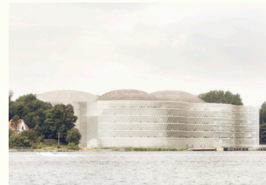
Process tanks and office space , 2012
