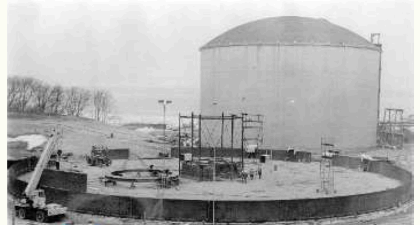
Construction of second silo , 1968
