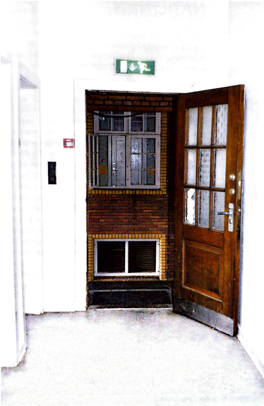
Fig. 1-11 Emergency exit, Randers Barracks. Credit: (Juhl, 2004, pp 23)
