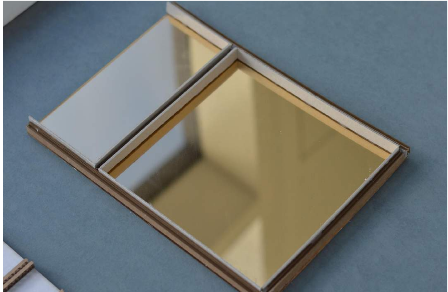
Double extruded frame with protrusion away from the facade plane.
