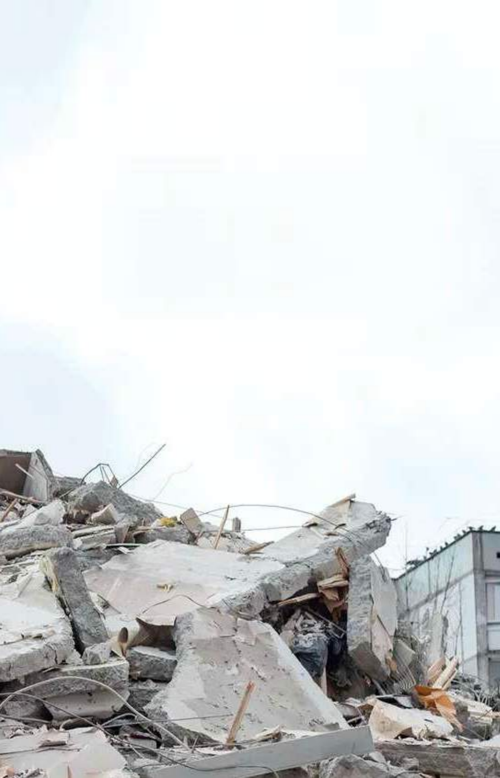
Demolished buildings adjacent to site.
