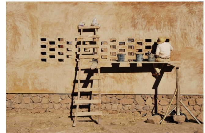
figure 27 | BC Architects Preschool of Ouled Merzoug Morocco
