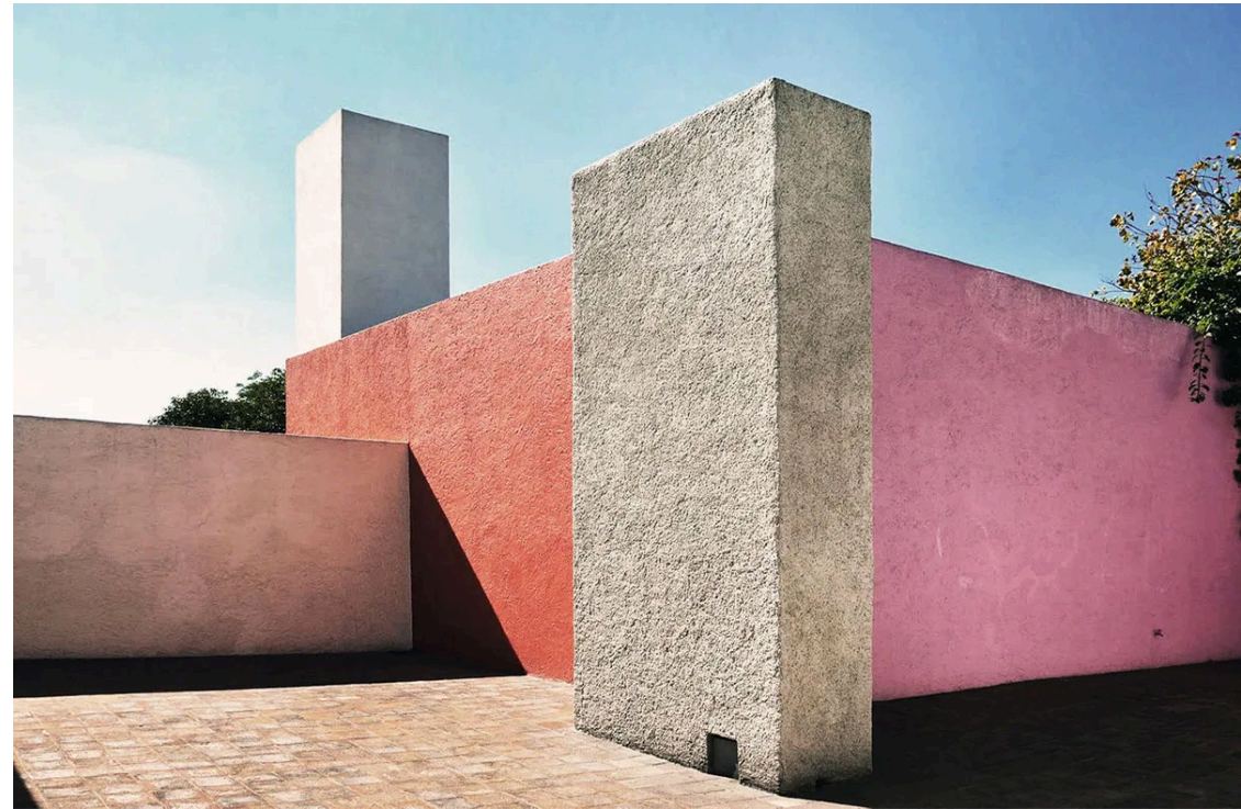
figure 25 | Casa Luis Barragán Mexico City, Mexico
